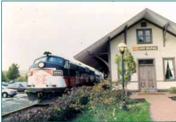
New Milford Train Station.
