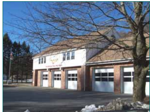
Northville Fire Station.
