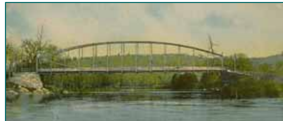
Boardmans Bridge, c. 1913.
