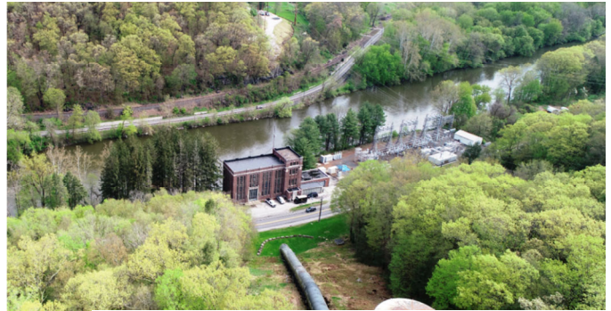
Rocky River Pumped Hydro Storage Station
