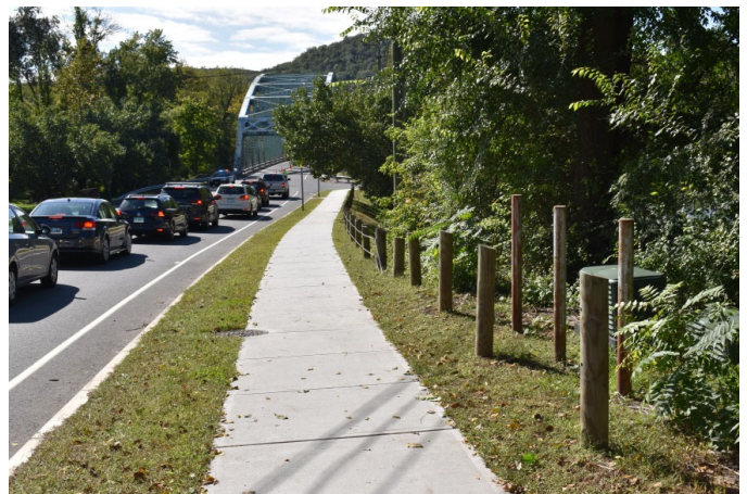
Newly reconstructed sidewalk along Bridge Street
