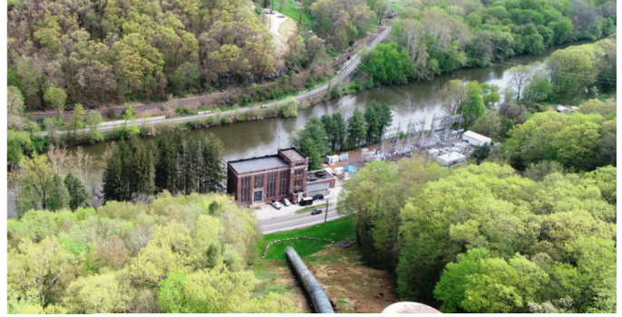
Rocky River Pumped Hydro Storage Station
