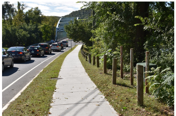
Newly reconstructed sidewalk along Bridge Street
