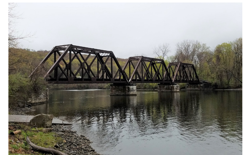
Existing Railroad Bridge at the Bleachery
