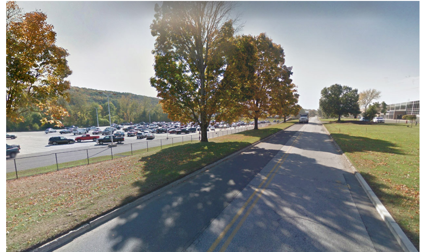
Existing Condition on Pickett District Road
