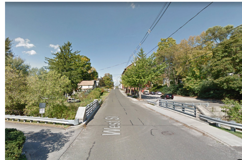
West Street Bridge Over Great Brook
