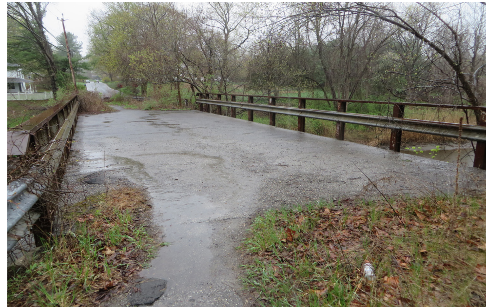
Existing Lanesville Drive Bridge
