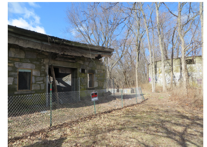
Existing Powerhouse and Storage Tank
