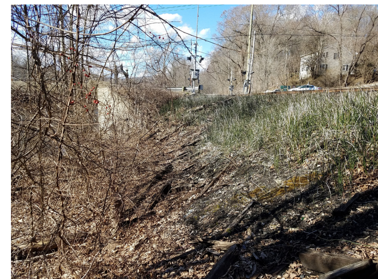
Existing Conditions in Vicinity of Boardman Bridge
