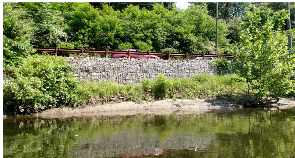
Existing condition looking from the river
