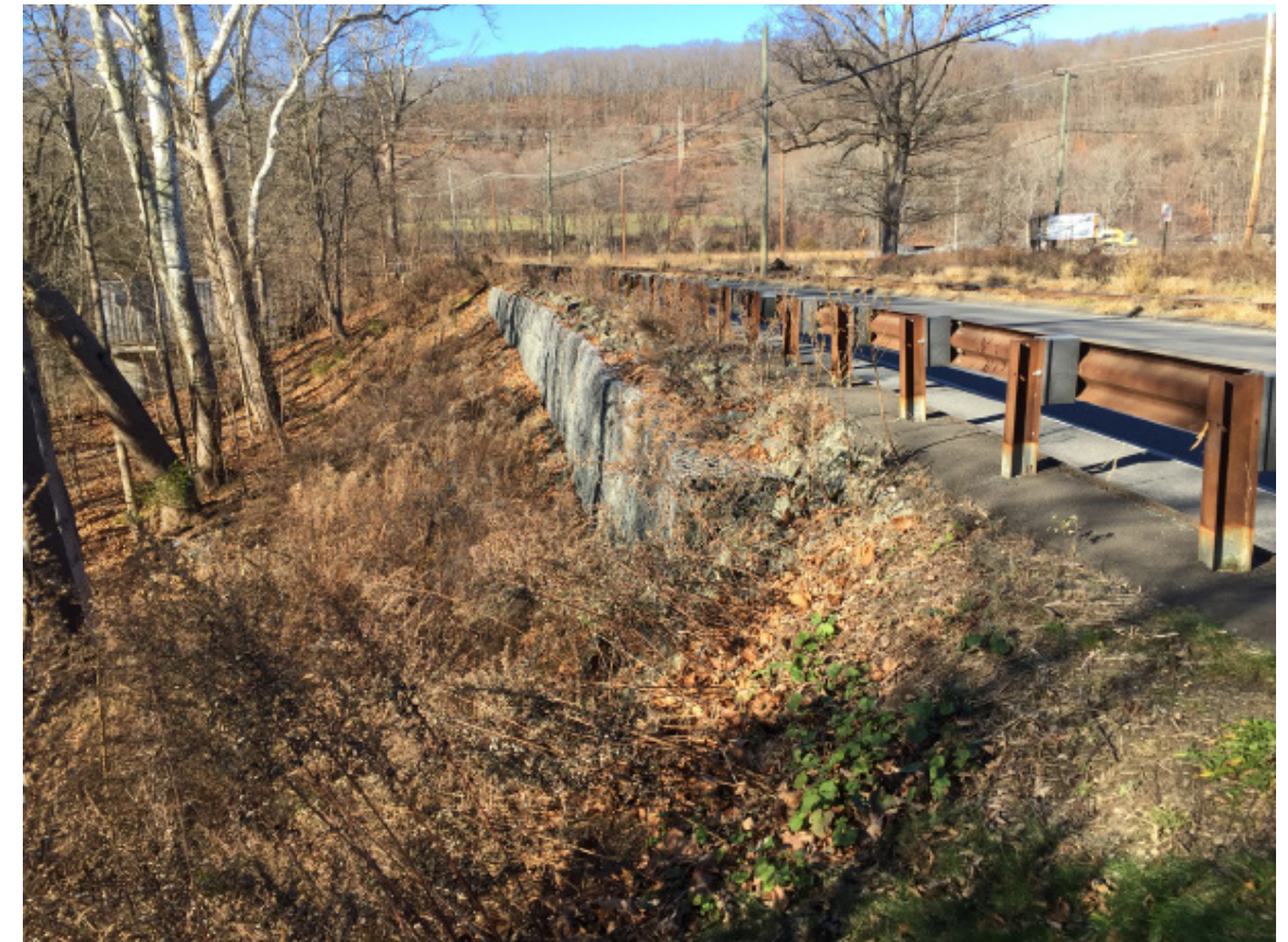
Existing Condition along Housatonic Avenue
