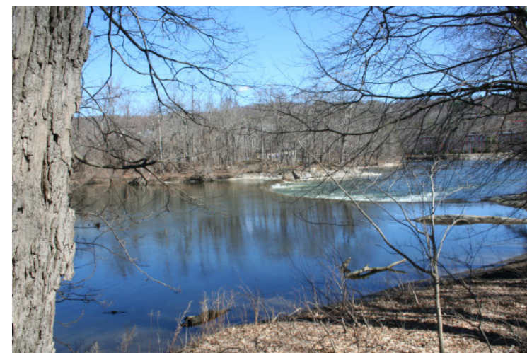
View Upstream of Dam in the Housatonic River
