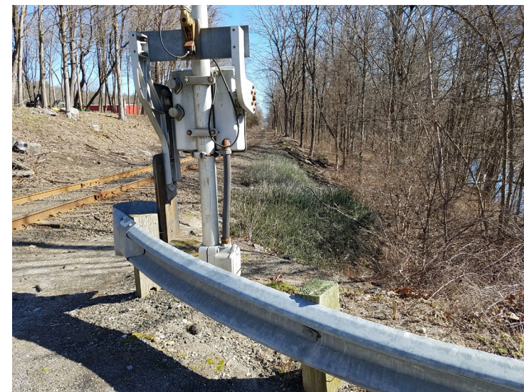
Existing crossing at Boardman Road
