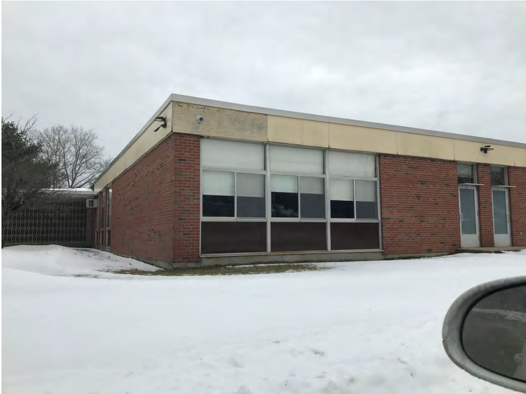
Building Exterior – West Elevation
