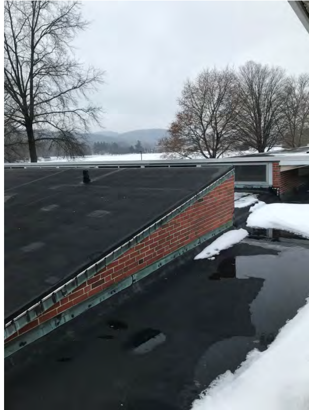
Example of rubber membrane roof and trough roof design
