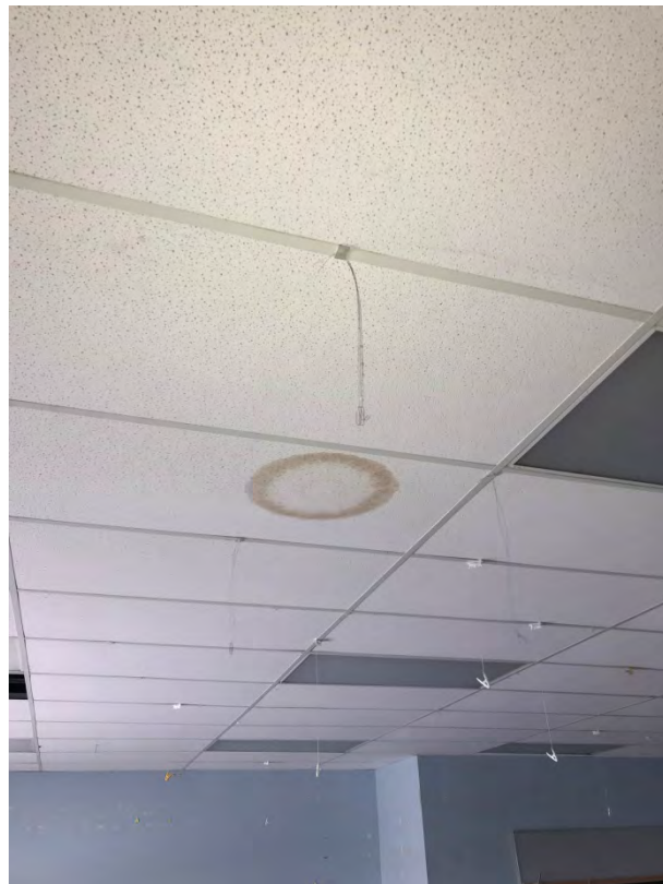
Example of typical water staining on ceiling
