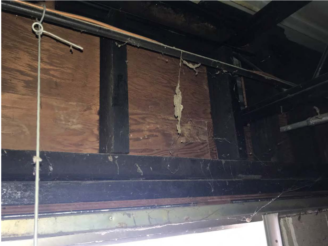
Assumed creosote treated wood
