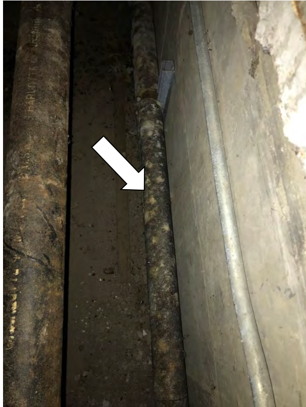
Mold impacted pipe insulation within pipe tunnel
