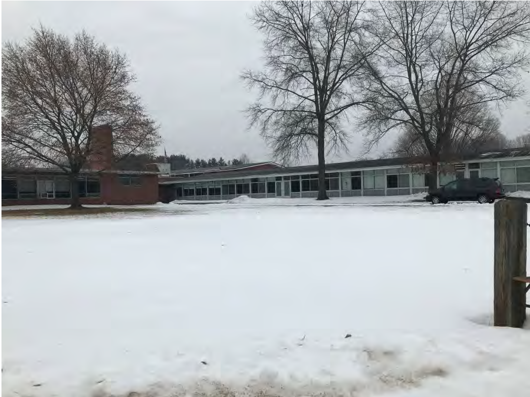
Building Exterior – East Elevation
