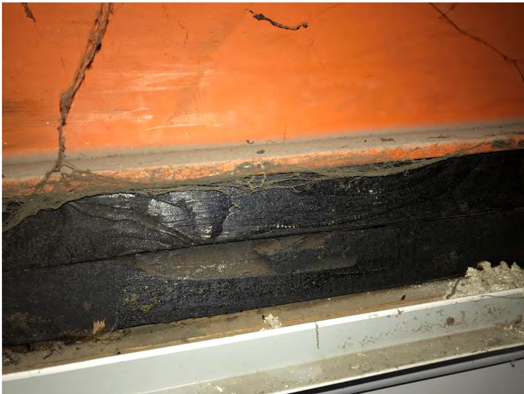
Assumed creosote treated wood
