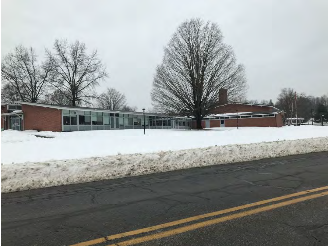
Building Exterior – North Elevation
