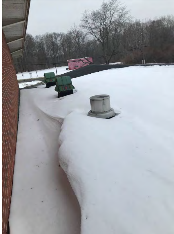
Exterior roof showing buildings exhaust points
