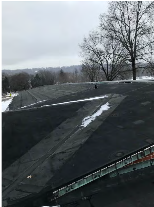
Example of rubber membrane roof
