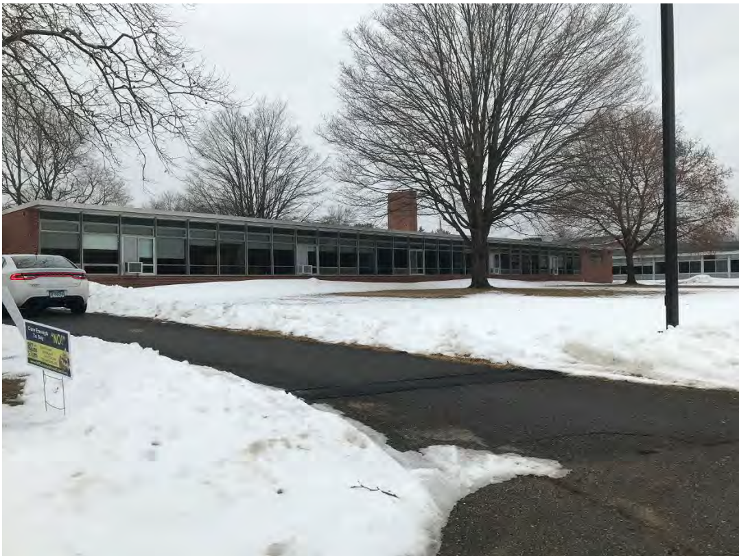
Building Exterior – East Elevation
