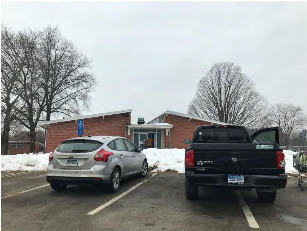
Building Exterior – East Elevation
