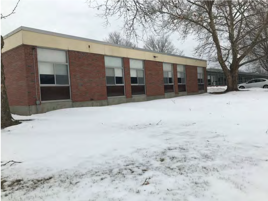
Building Exterior – East Elevation
