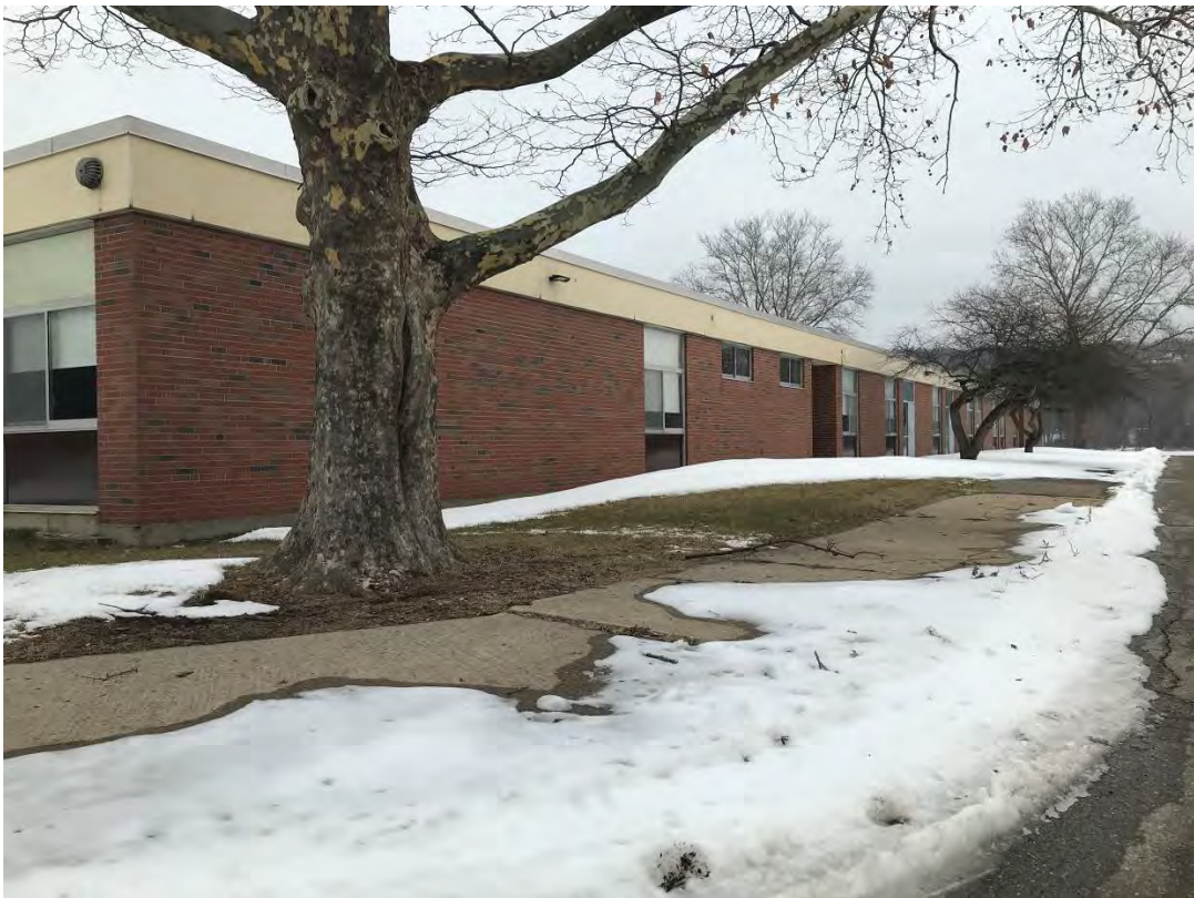
Building Exterior – South Elevation
