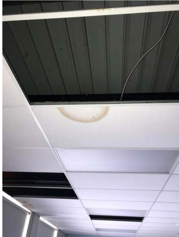
Example of typical water staining on ceiling
