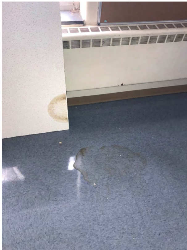
Example of typical water staining on floor
