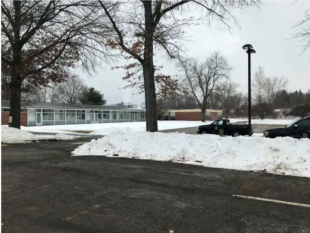
Building Exterior – West Elevation
