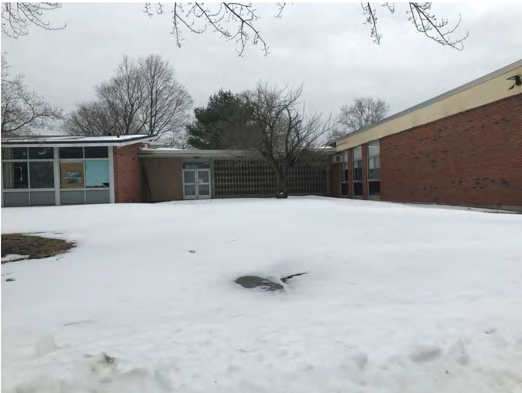
Building Exterior – West Elevation
