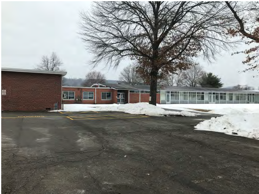
Building Exterior – West Elevation
