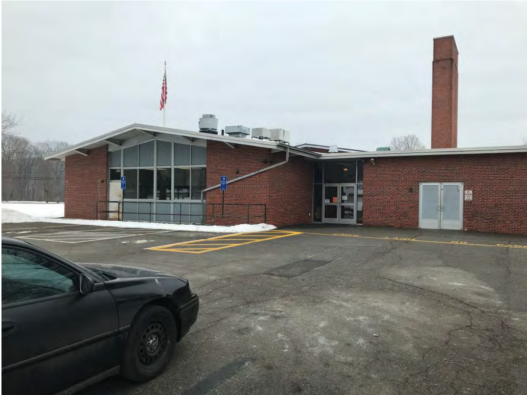
Building Exterior – West Elevation
