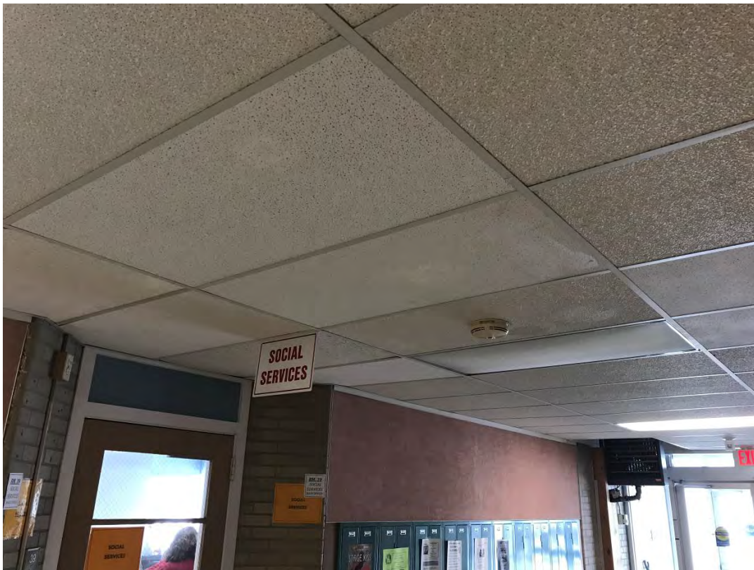
Example of water damaged ceiling tiles that have been painted
