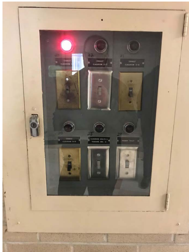
Room exhaust fan control box (two are present in the building)
