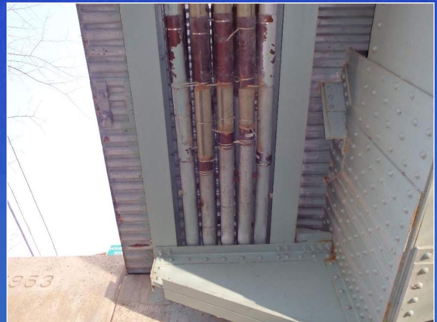
Communication Conduits – North Fascia
