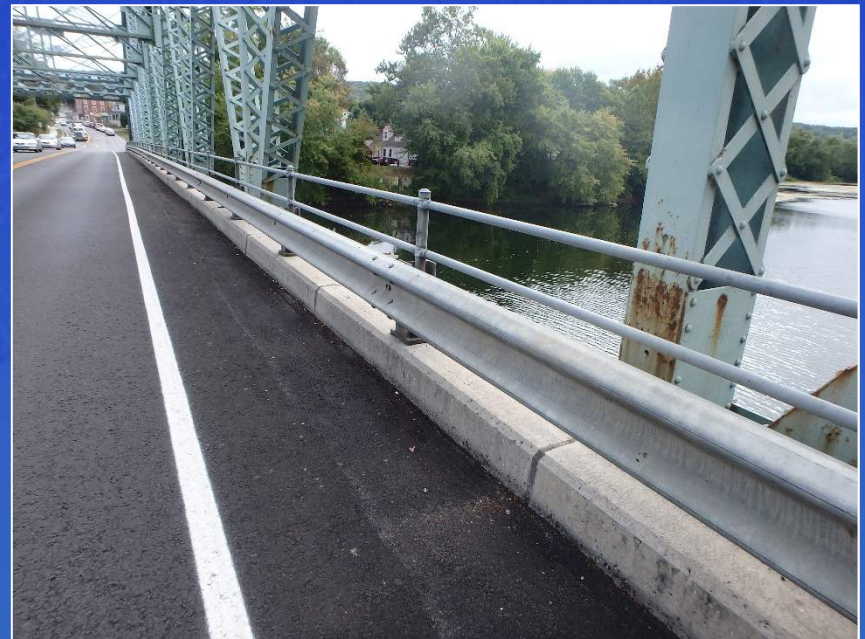
Typical Bridge Curb and Railing
