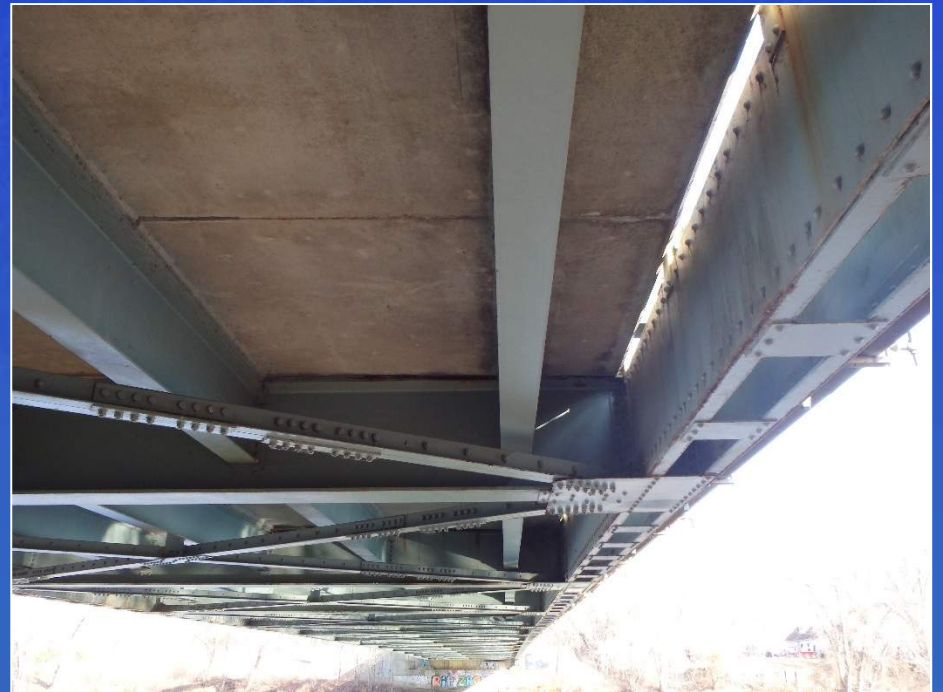
Typical Underside of Deck and Truss
