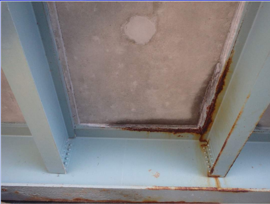
Typical Leaking at Deck Panel Joints Note: Active Rust on Stringer and Beam
