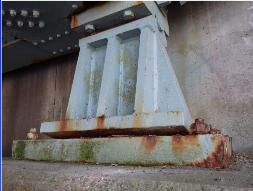
Typical Rocker Bearing (West Abutment)
