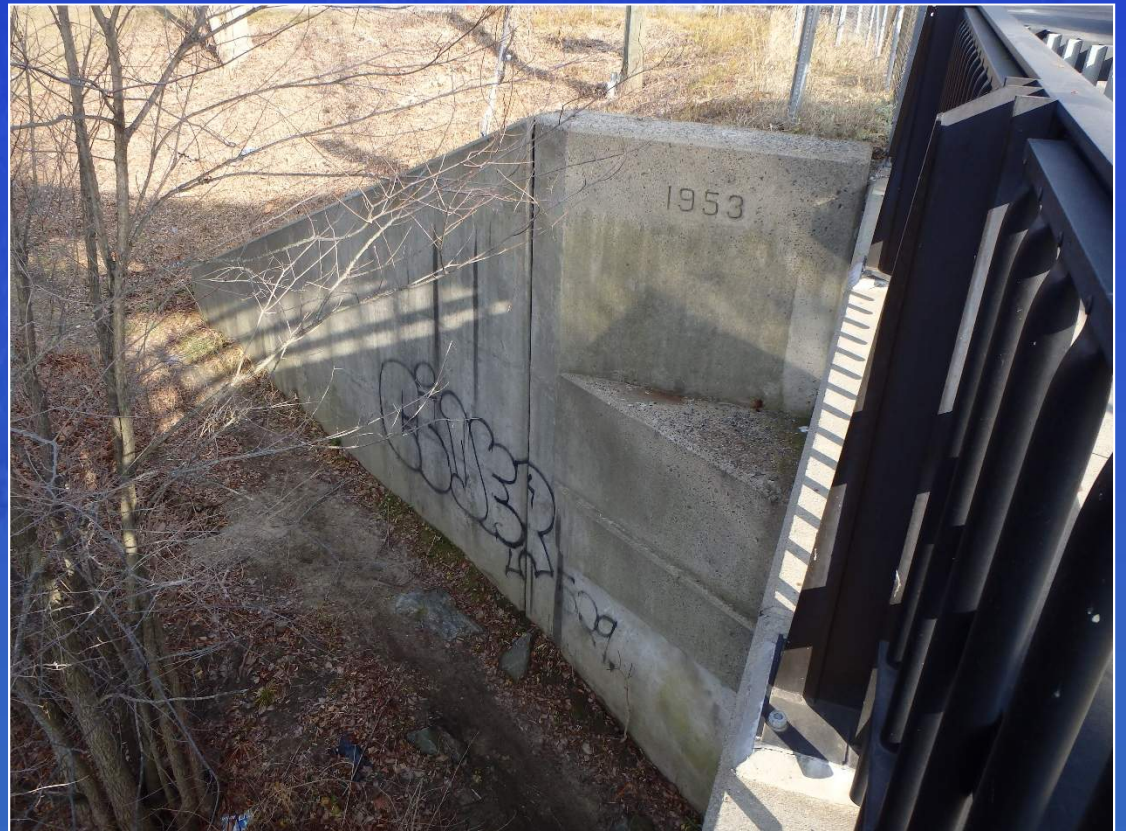
Northeast Wingwall (Typical)
