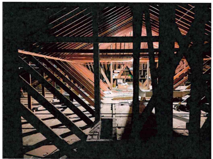
Attic roof construction – wood rafters & wood decking
