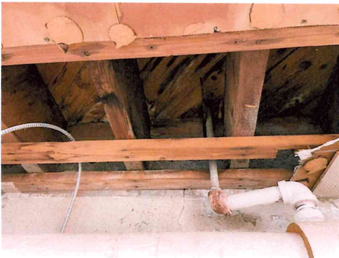
Typical floor joist construction bearing on perimeter masonry
