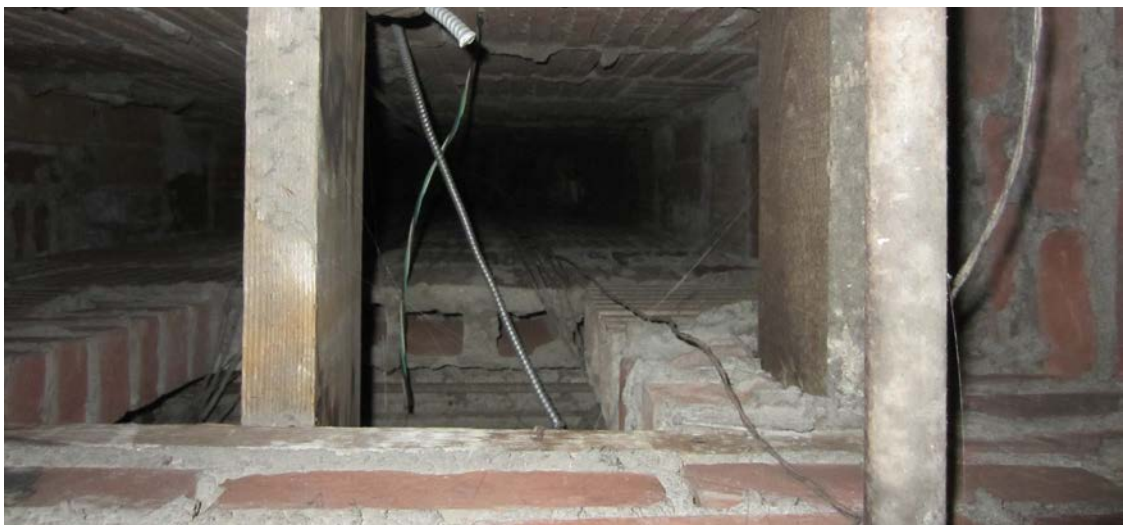
Convection Air Shafts
