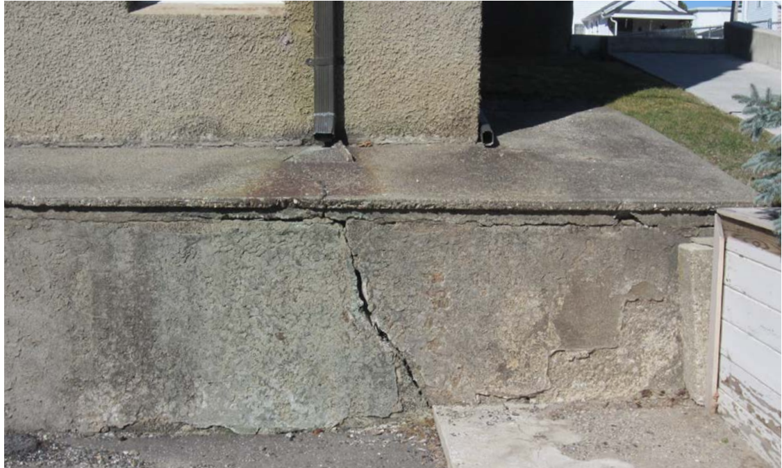
Crack in Steam Tunnel
