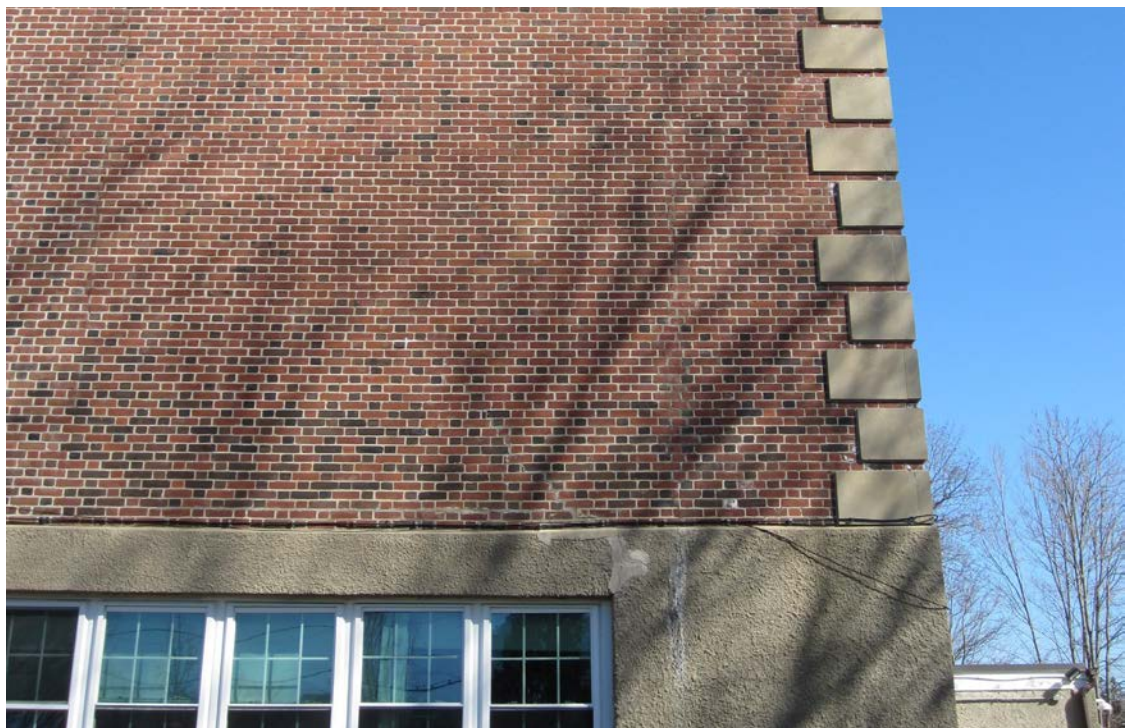
Cracks in Brickwork on South Facade
