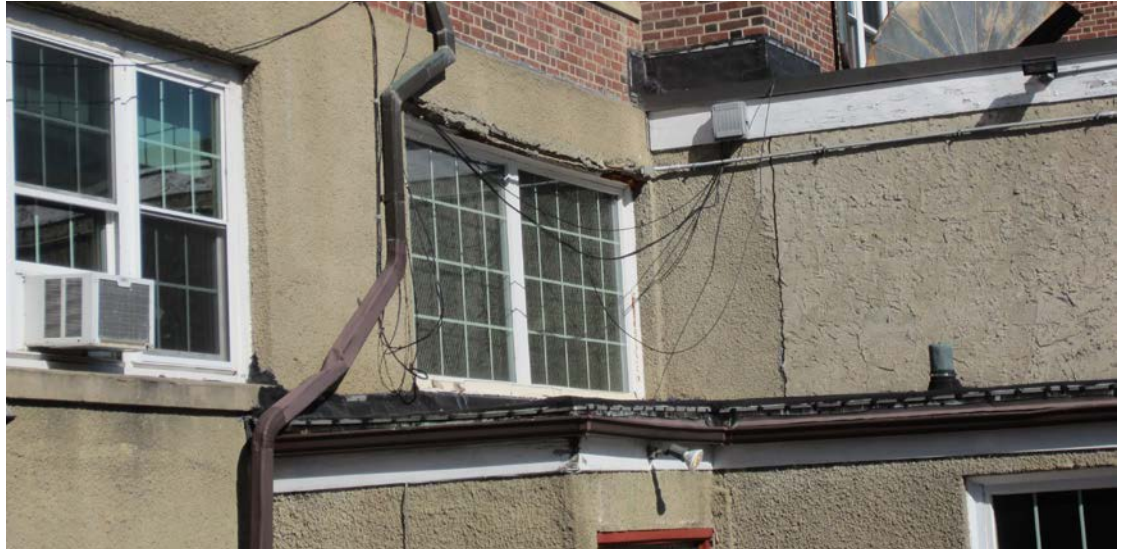
Rusted Steel Lintel
