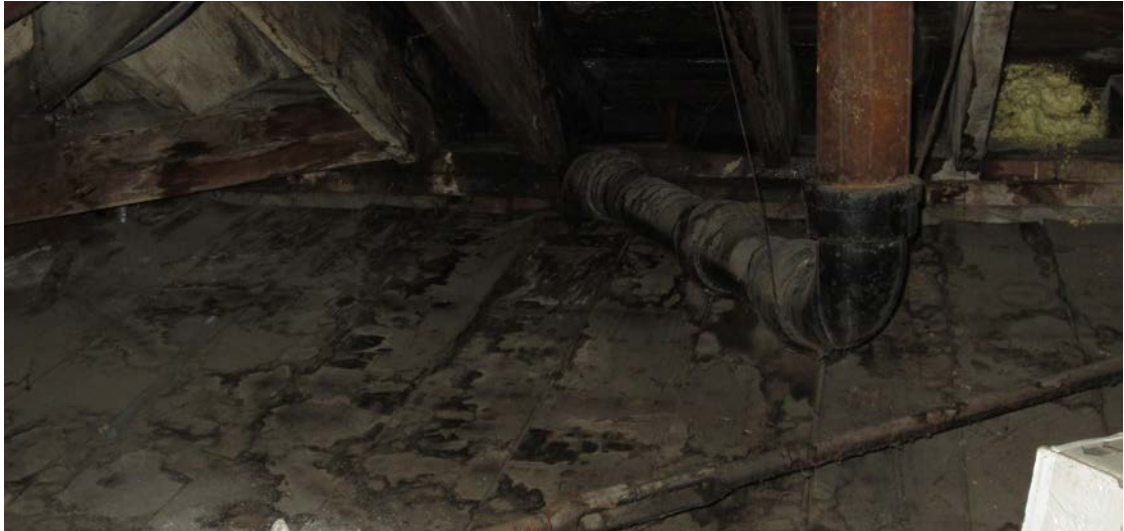
Water Damage Visible in Attic
