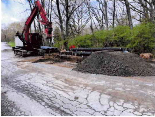
April Dr. drainage pipe replacement
